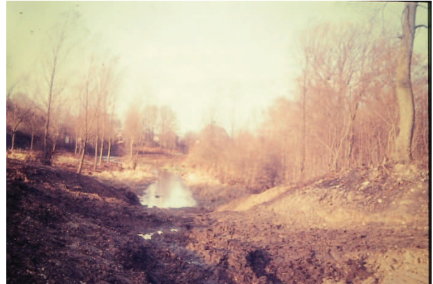
Digging out the moats 1971
